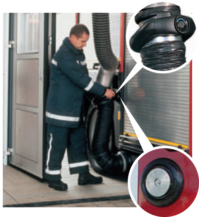
The anchor plate is the nozzle attaching point on the vehicle. It is mounted at a convenient height on the vehicle body enabling you to attach the nozzle while standing up right. The electro-magnet has an ergonomic handle and attaches instantly to the anchor plate on the vehicle.
